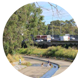
2 Concrete Lined Gardiners Creek (KooyongKoot) Highly modified and urbanised creek, to facilitate water management for the catchment. Sections of the creek were lined with concrete to increase water capacity.
