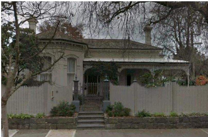
Figure 10. 11 Avondale Road, Armadale (Significant in HO123). (Source: Google Streetview).
