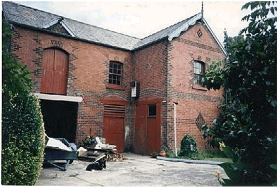
Figure 11. Stables at 14 Sorrett Avenue, Malvern (HO396) (source: National Trust, nd).
