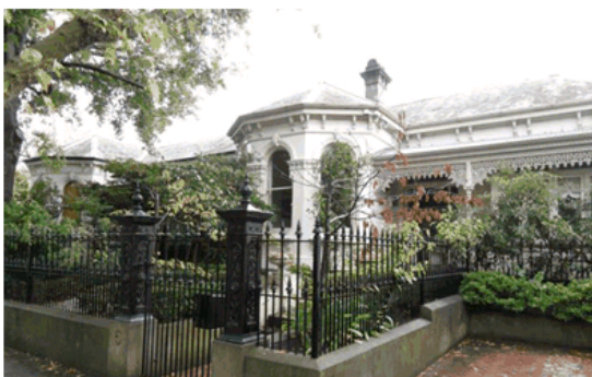
Figure 2 Villas 3 (left) and 5 (right) Avondale Road Armadale
