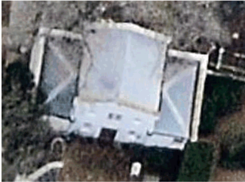
Figure 7. Oblique aerial view of the stables at 3 Avondale Road. (Source: NearMap.com, August 2016)
