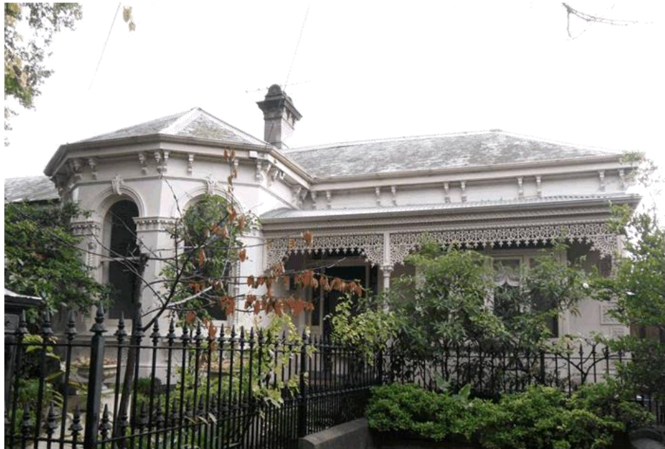
Figure 4. Front façade of 5 Avondale Road. Note casement box bay window beneath verandah. (Source: Context, 2017)
