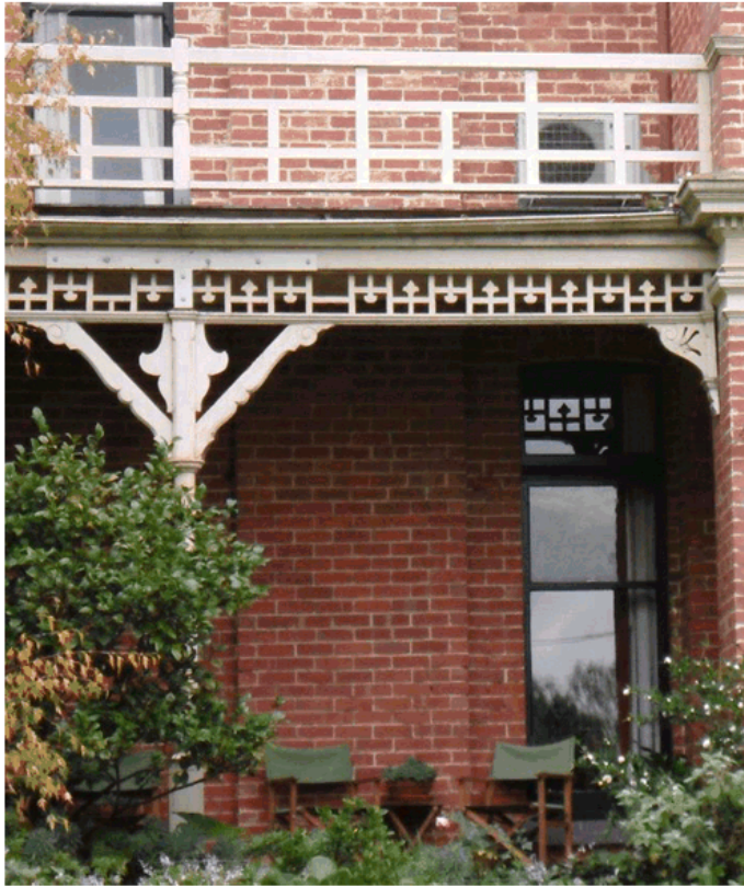
Figure 6. Detail of the verandah and balustrade. (Source: Context, 2017)
