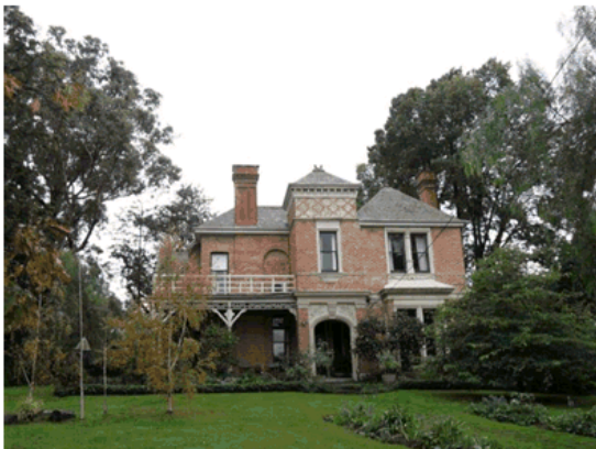
Figure 1 17-19 Ethel Street, Malvern
