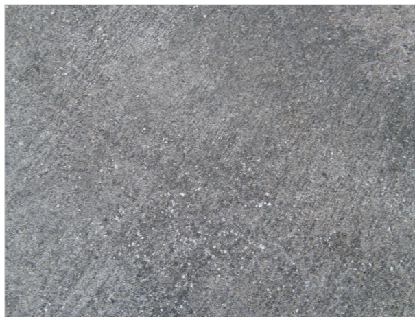
REN1 - CONCRETE RENDER RENDER OVER EXISTING CONCRETE COLUMNS & UPSTAND - WEST WALL
