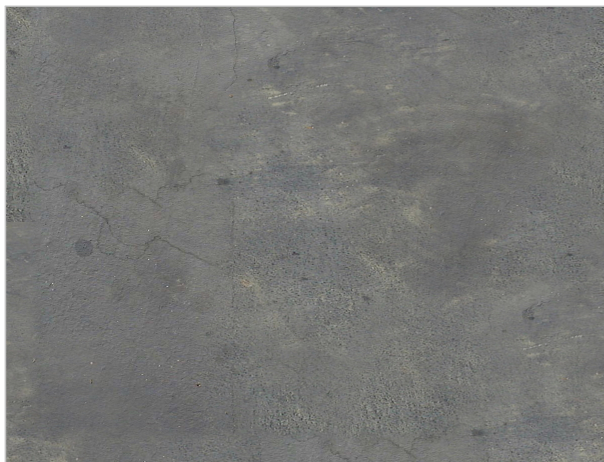
FCO - CONCRETE SLAB & STAIRS ENTRY STAIRS & WALKWAY
