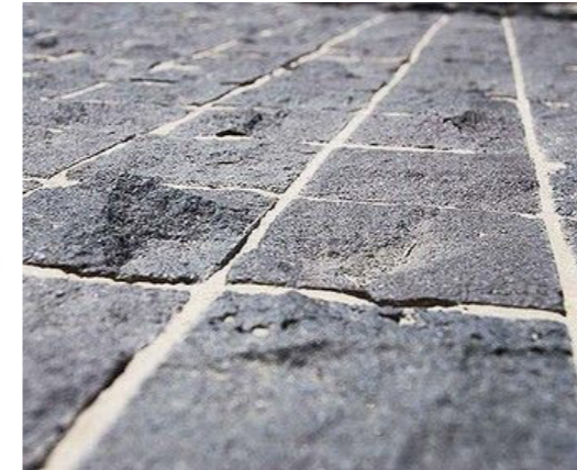
Bluestone Feature Paving
