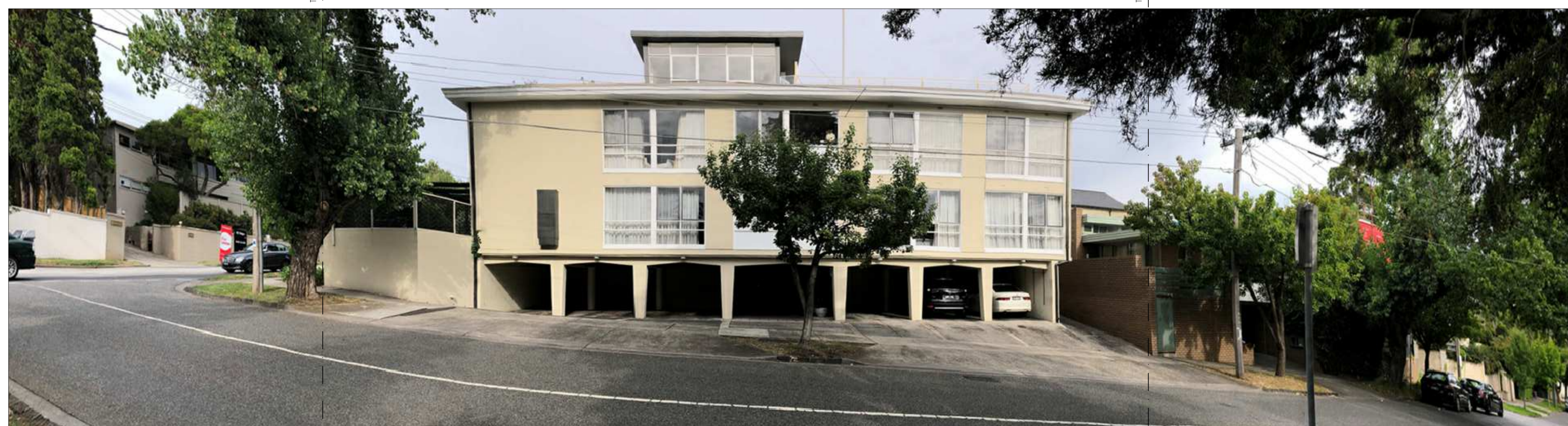
EXISTING STREETSCAPE - MOONGA ROAD
