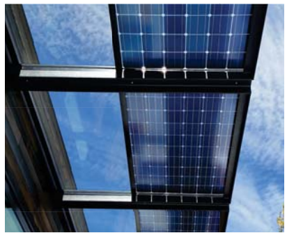
② Bifacial PV As Horizontal Screen Device and pergola structure
