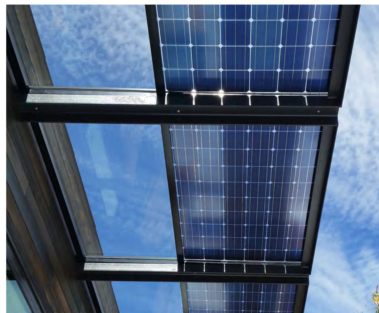
2 Bifacial PV As Horizontal Screen Device and pergola structure
