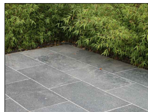
LANDSCAPING - BLUESTONE PAVING
