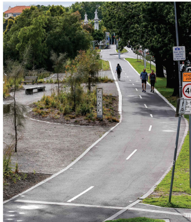
Shared Path - Asphalt with concrete edge
