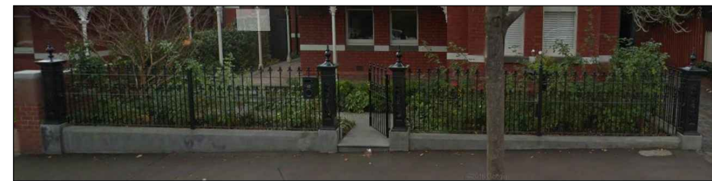
EXAMPLE OF PROPOSED 5 EVELINA ROAD BOUNDARY FENCE. BLACK STEEL PICKETS ON RENDERED CONCRETE BASE. MAX. HEIGHT OF 1.2m, SLIDING VEHICLE GATE AND SWING PEDESTRIAN GATE.
