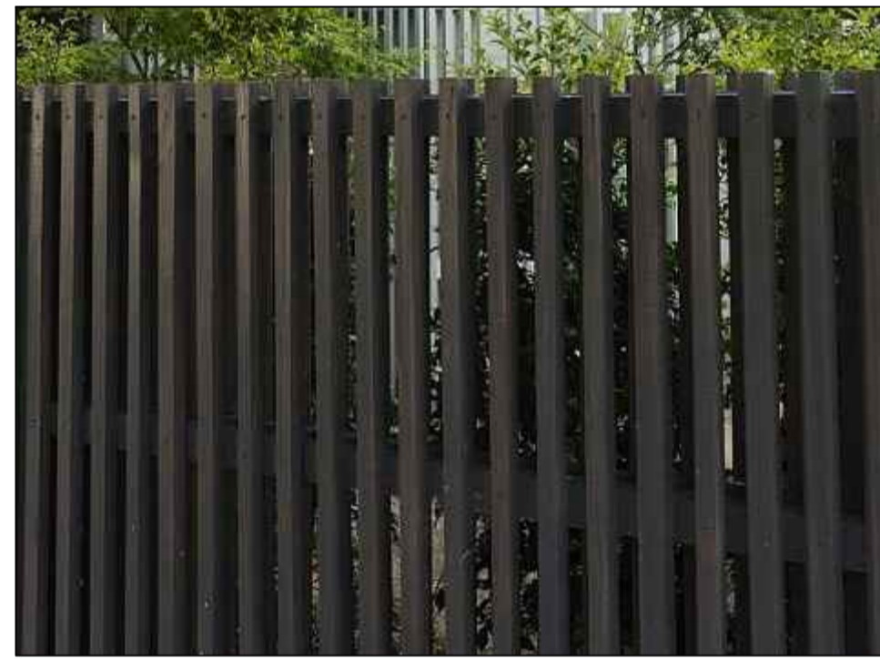
TIM-01 TIMBER BATTENS BACKED BY SOLID PANELS
