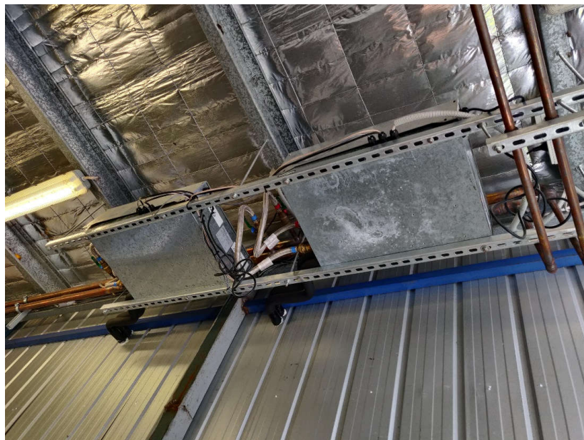
TCR 2 (Mechanical plant located inside shed)
