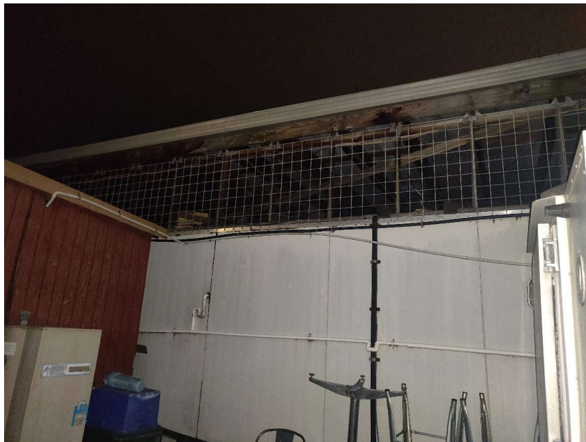
OCR 3 (Mechanical plant located inside shed)
