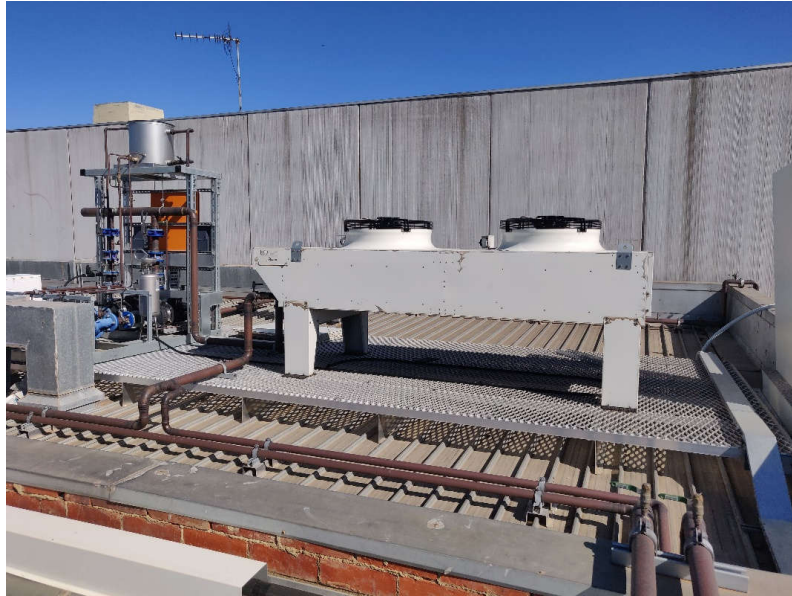
TCR 1 (Mechanical plant located above store)
