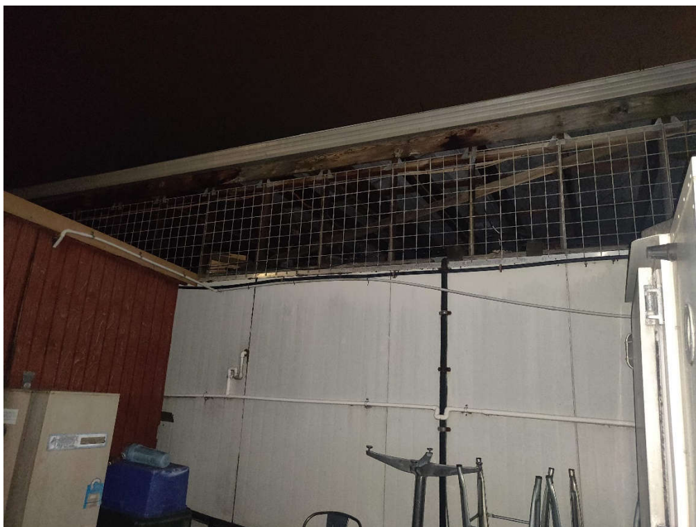
OCR 3 (Mechanical plant located inside shed)
