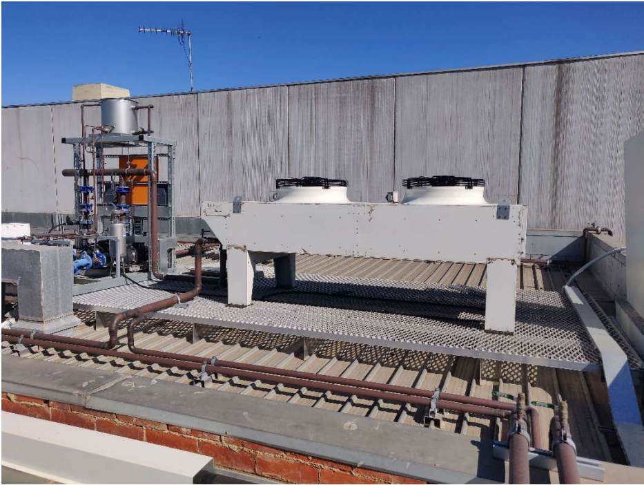
TCR 1 (Mechanical plant located above store)
