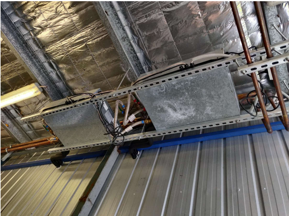
TCR 2 (Mechanical plant located inside shed)
