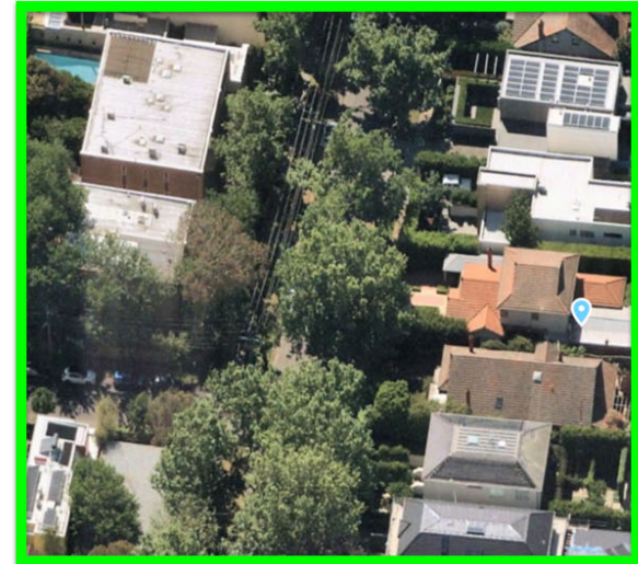
Eastern Elevation (view towards Glenferrie Road)
