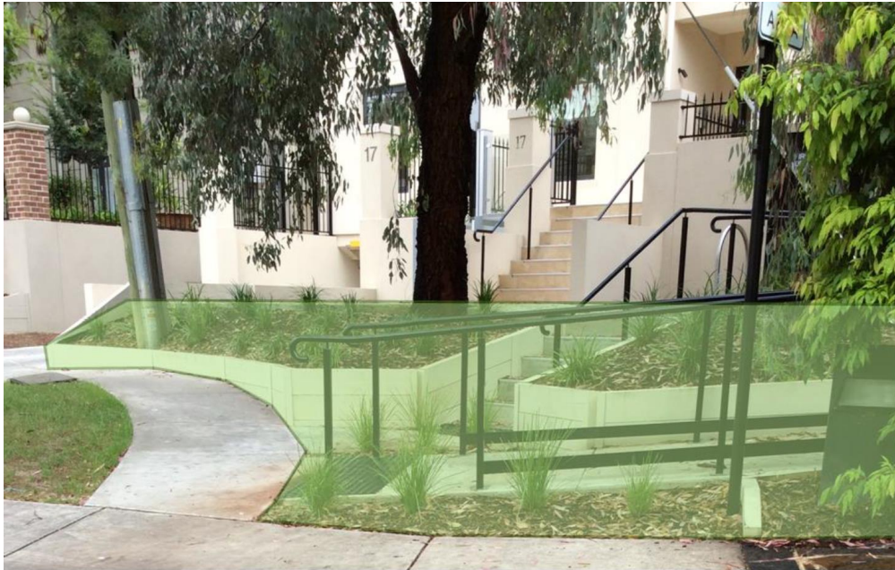
Figure 3. Disabled Ramps, steps and landscaping built on Council road Reserve
