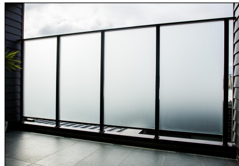
BA.02 Glass Balustrade Obscure OG Obscure Glass to 1.7m above FFL PS.01 Privacy Screen - Obscure Glass to 1.7m above FFL
