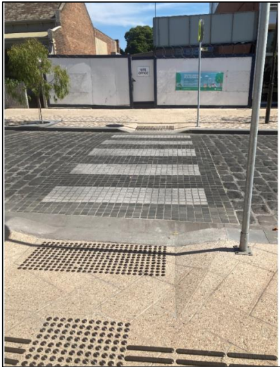
Figure 4.2 Zebra crossing along Izett Street, Prahran
