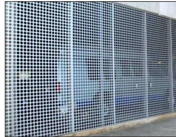
MF.02 Perforated metal car stacker sliding doors powder-coated 'White'
