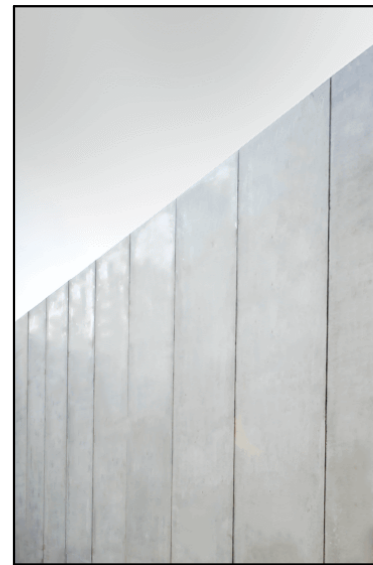
CP.01 Precast concrete panel 'Natural finish'
