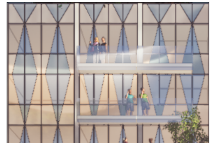
GL.02 Glass Curtain Wall - 'Diamond' Bronze and Blue glass - 'Charcoal' frame
