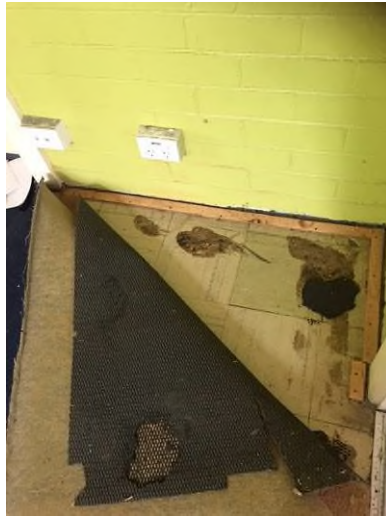
Photograph 3: Stairs/Foyer- Asbestos vinyl floor tiles below carpet
