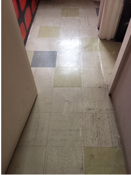
Photograph 1: Toilet – Asbestos vinyl floor tiles
