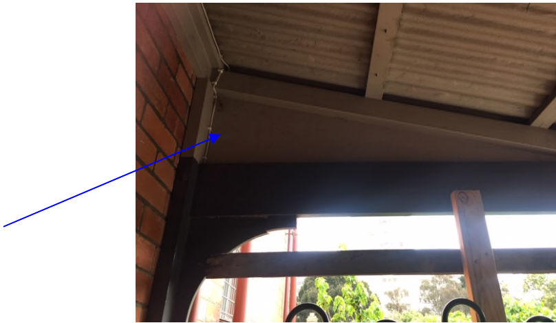
Photograph 4: External- Asbestos cement sheeting
