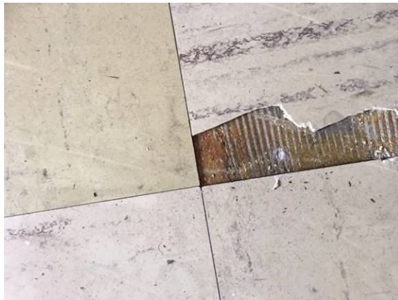
Photograph 2: Kitchen- Asbestos vinyl floor tiles
