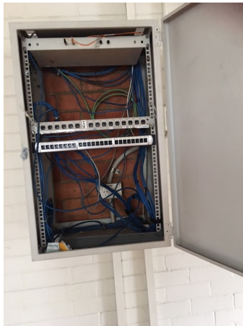
Photograph 7: Open space- No electrical switchboard noted in cupboard
