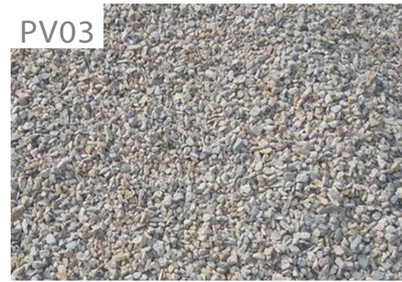
Paving type 03 - compacted toppings surface
