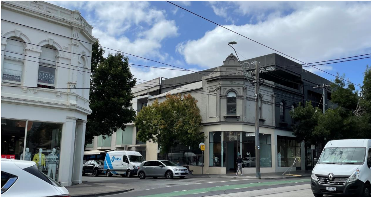
Figure 6 566 Chapel Street (at right of intersection), with 568-70 Chapel Street at left
