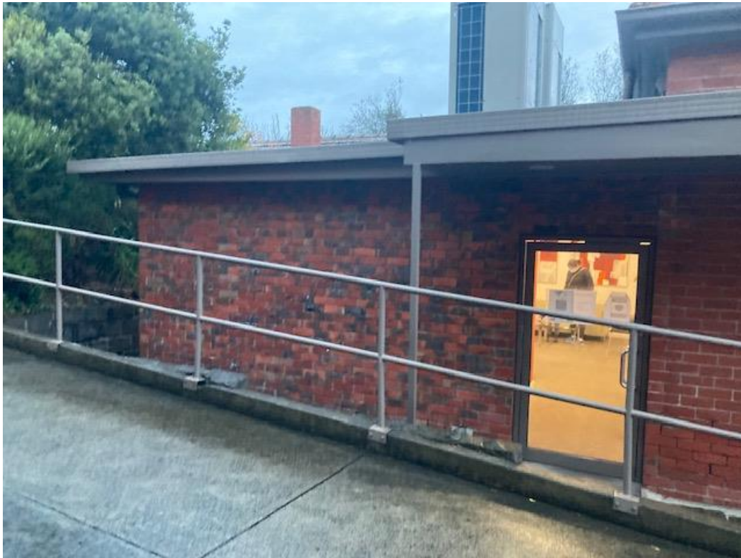
Figure 7 – The north entry and rear of the subject house (Belinda Minc)
