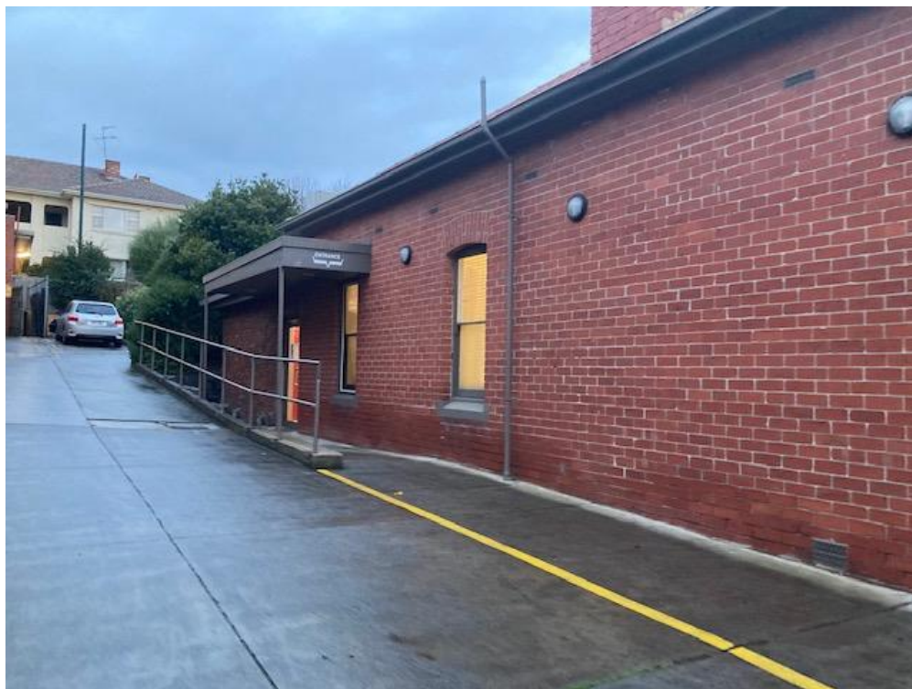
Figure 6 – The north side of the subject house (Belinda Minc)
