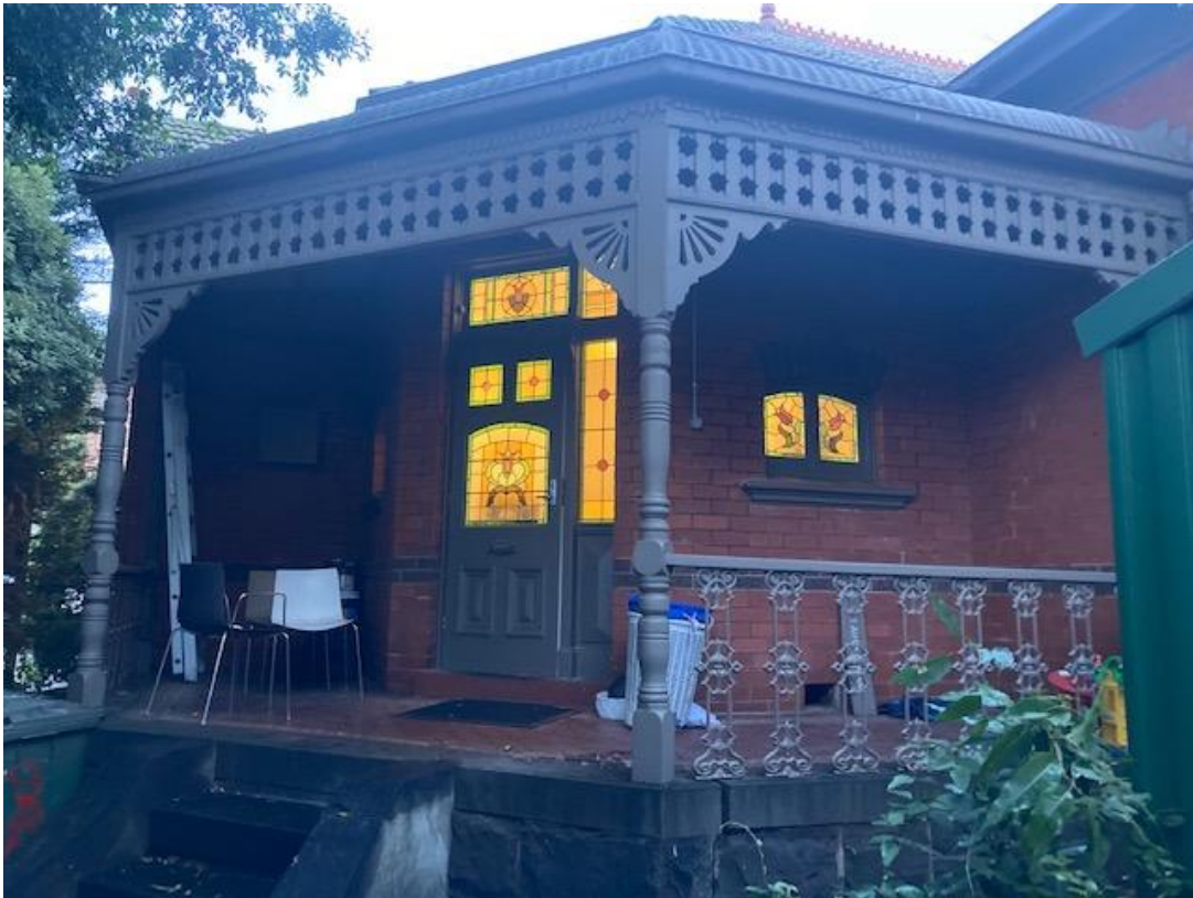
Figure 3 – Front entry to the subject house
