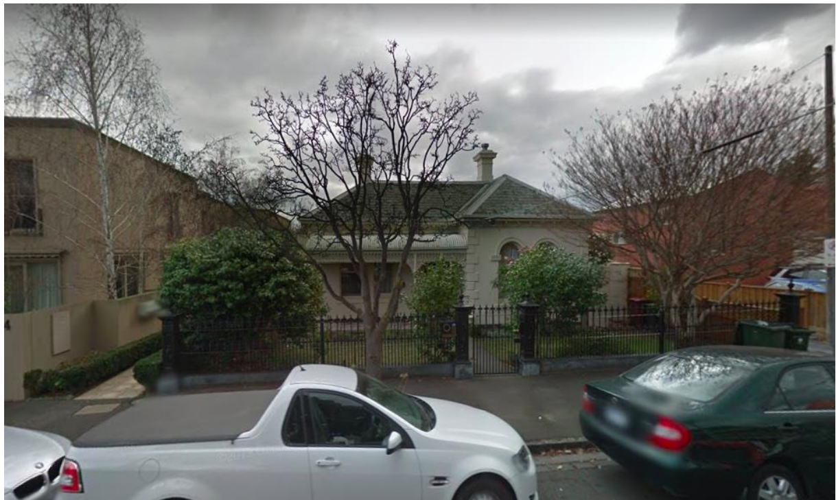
Figure 10 – 2 Airlie Avenue, Prahran (Google Streetview)
