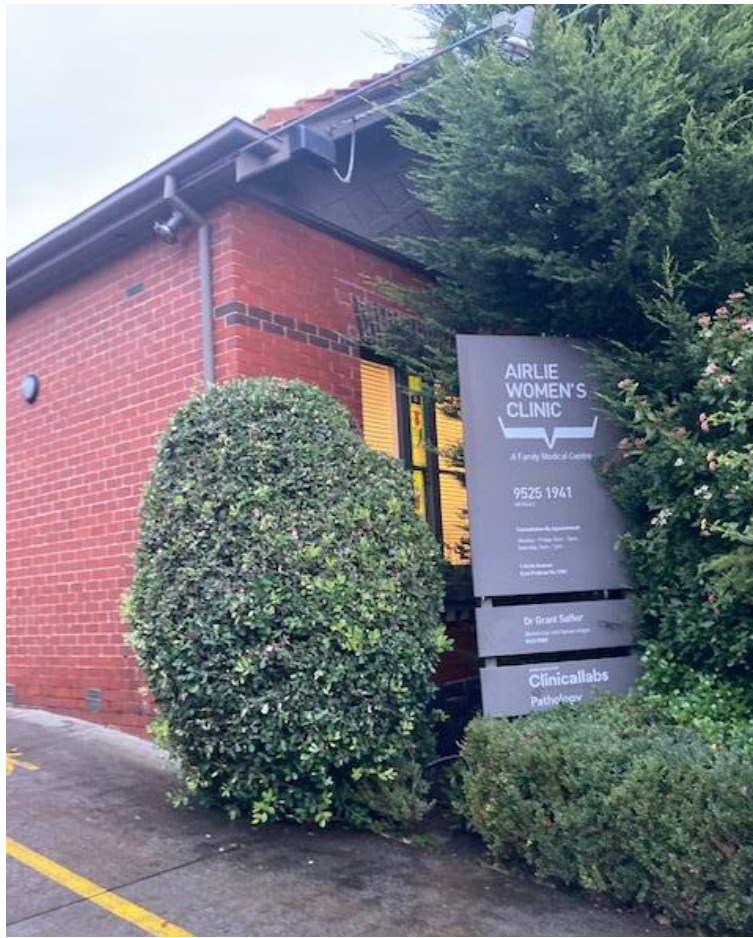
Figure 5 – The subject house from the north side
