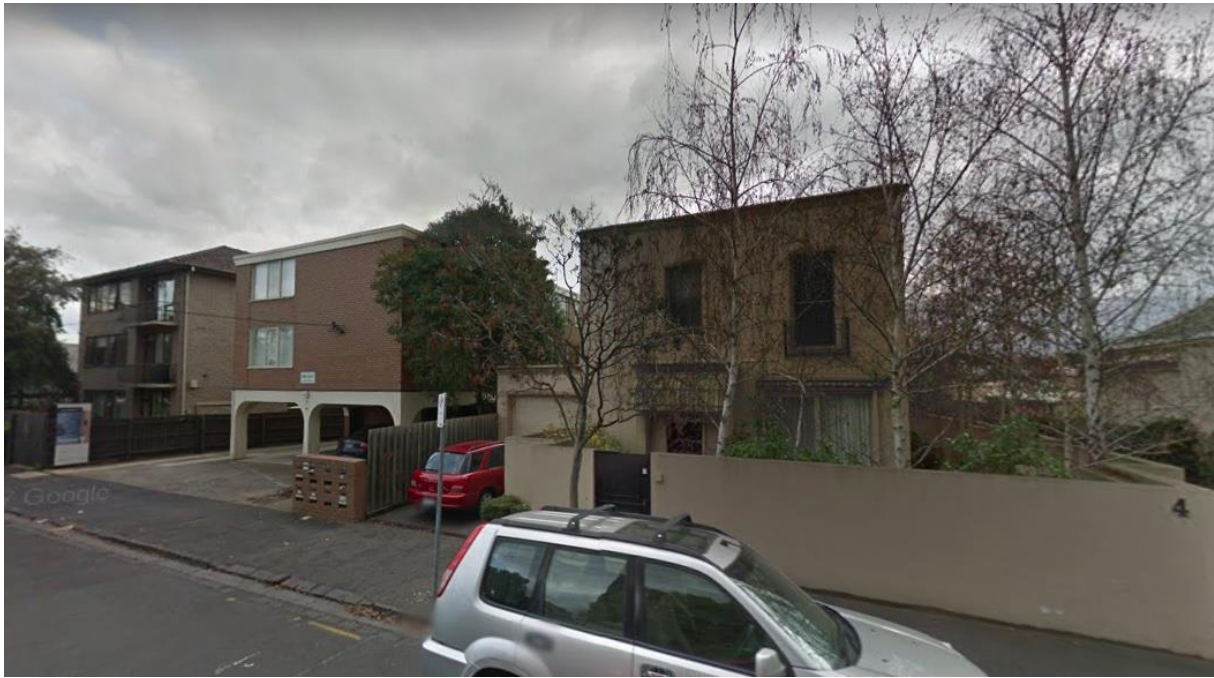
Figure 11 – 4, 6 & 8 Airlie Avenue, Prahran (Google Streetview)
