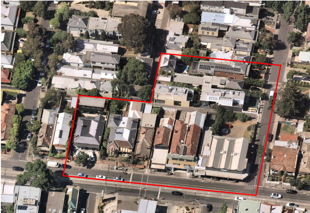
Figure 15 Aerial photograph with nos 546-576 High Street and 96-100/100A Chomley Street indicated Source Nearmap, downloaded 27 September 2021
