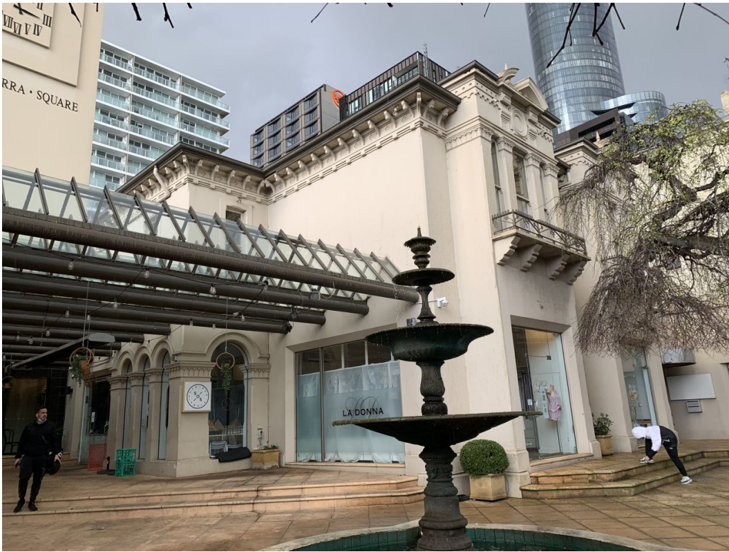
Figure 13 South and west elevations of 185-187 Toorak Road, showing new openings to ground level and classical detailing to the upper levels
