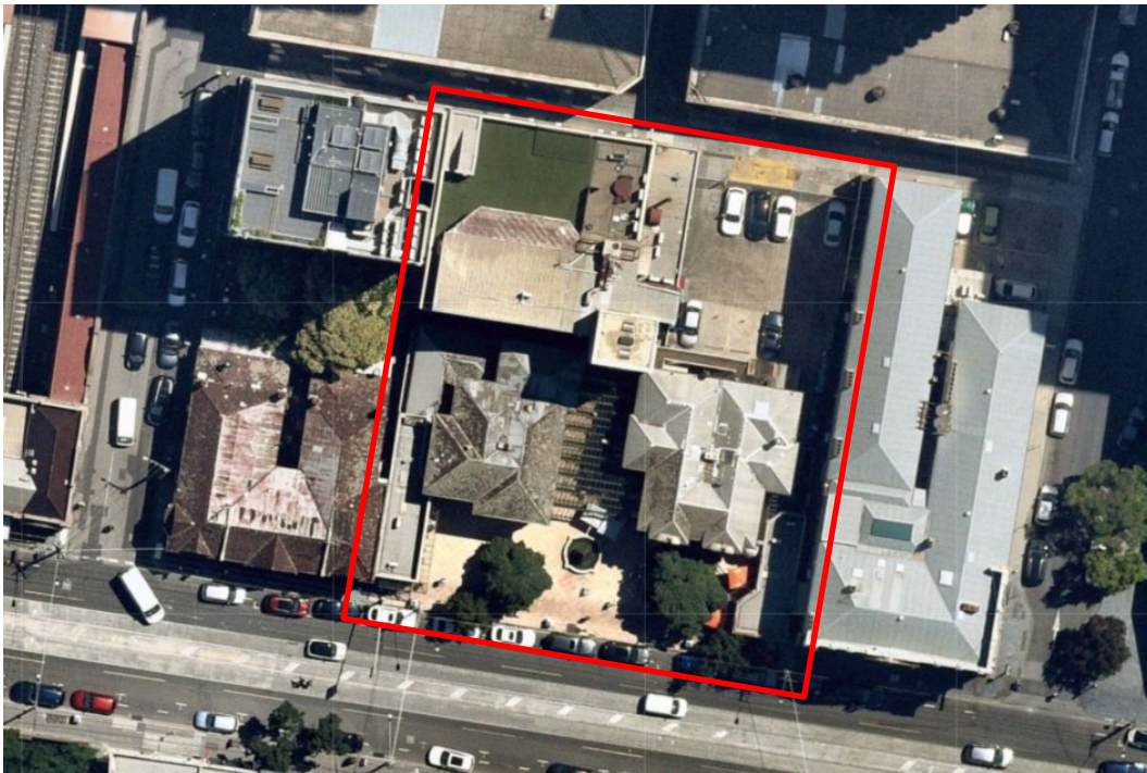
Figure 8 Recent aerial photograph of the subject site Source: Nearmap, January 2021
