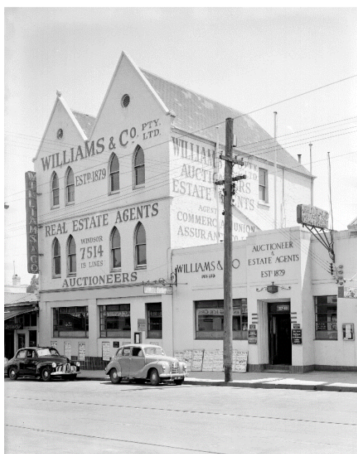
Figure 10. Williams & Co Estate Agents premises at 155-157 Toorak Road c.1950. (Source: Lyle Fowler, SLV)
