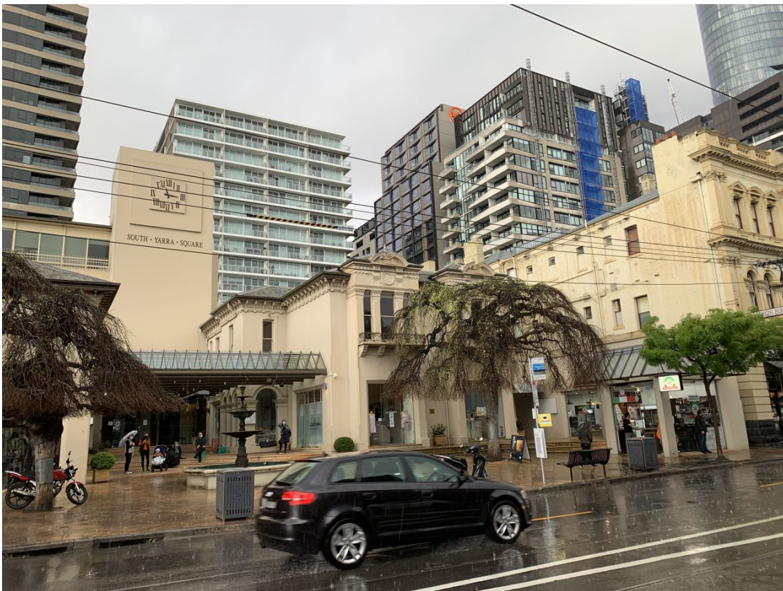
Figure 12 View of the subject site showing 185-187 Toorak Road, the plaza and newer development to the eastern boundary
