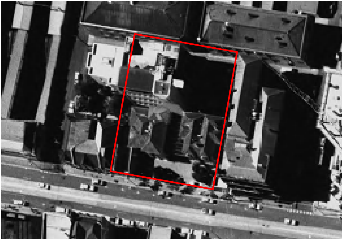
Figure 24 Aerial photograph from 1984, showing the carpark to the north-east of the site following the demolition of the rear wings to 185 and 187 Toorak Road Source: Landata, Victorian Land Registry Services, Historical Aerial Photography Collection
