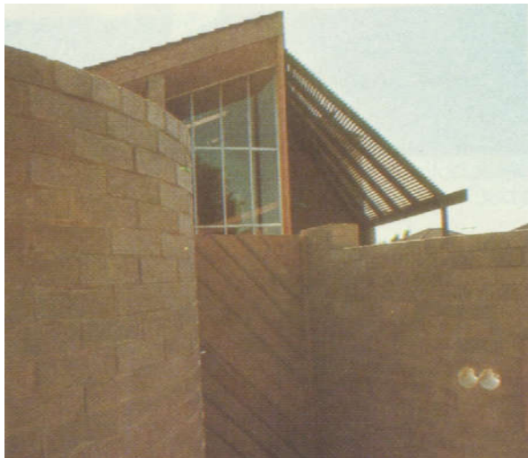
Figure 5: Another early view of the street frontage of the Crossman House Source: Belle , July/August 1978
