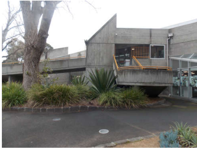
Figure 14: Harold Hold Memorial Swimming Pool, by Kevin Borland & Daryl Jackson in association (1966-69) Source: photograph by Built Heritage Pty Ltd
