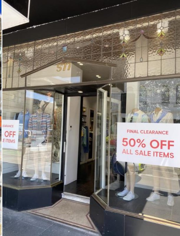
Figure 13. Intact interwar shop front at 577 Chapel Street, South Yarra with tiled ingo, original metal framed window, highlight window with leaded glass and tiled stall boards. (Source: Context, February 2020).
