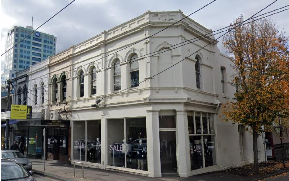
Figure 7. Row of five Victorian Italianate shops at 568-574A Chapel Street, South Yarra, built c.1891. (Source: Context, February 2020)
