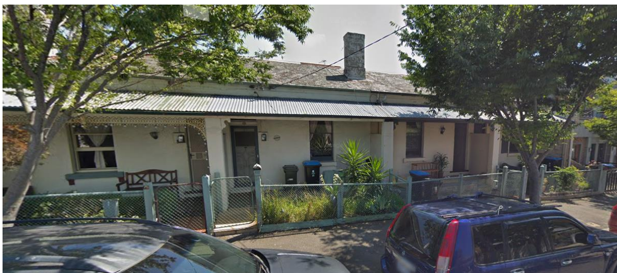
Figure 9. Terrace row at 19-25 Palermo Street, South Yarra are the earliest houses in the precinct, built c.1876. (Source: Google, January 2019)
