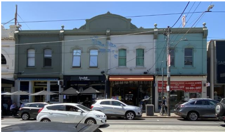
Figure 5. Victorian Italianate shops at 586-592 Chapel Street, South Yarra, built c.1890. (Source: Context, February 2020)
