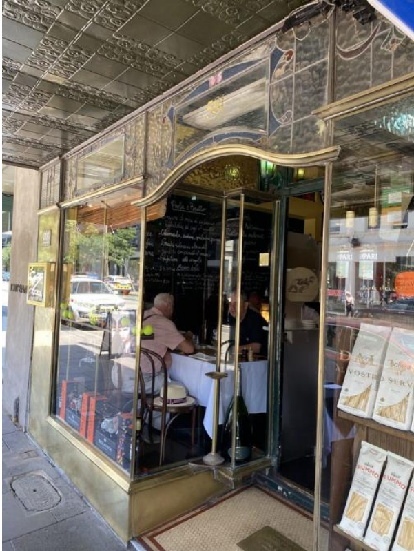
Figure 12. Intact Interwar shop front at 581 Chapel Street, South Yarra with tiled ingo, original metal framed window, highlight window with leaded glass and tiled stall boards. Of particular note is the Art Nouveau pressed metal soffit lining to the awning. (Source: Context, February 2020)
