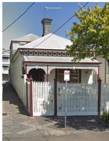
Figure 8. Typical example of a freestanding ashlar block fronted timber Italianate cottage. (Source: Google)
