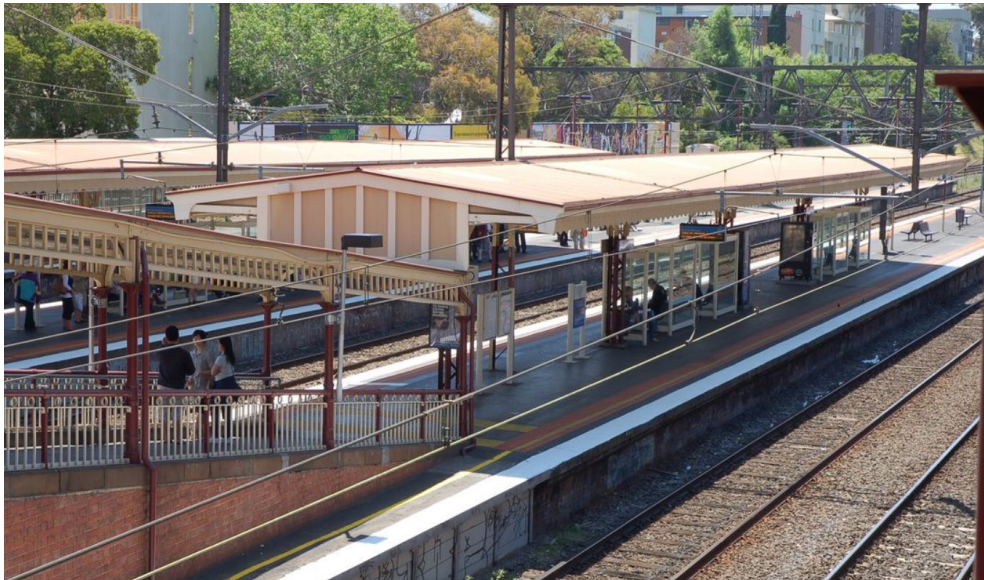
Figure 26. Covered ramp leading to platform with cantilevered canopy at the 'new' South Yarra Station (Source: film.vic.gov.au)
