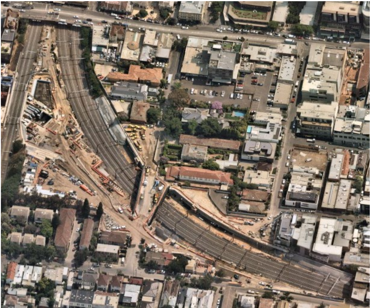
Figure 14. Aerial image showing the impact of Metro Tunnel works on the landscaped South Yarra Sidings and the removal of Lovers Walk between Toorak Road and Chapel Street. (Nearmap 2020)
