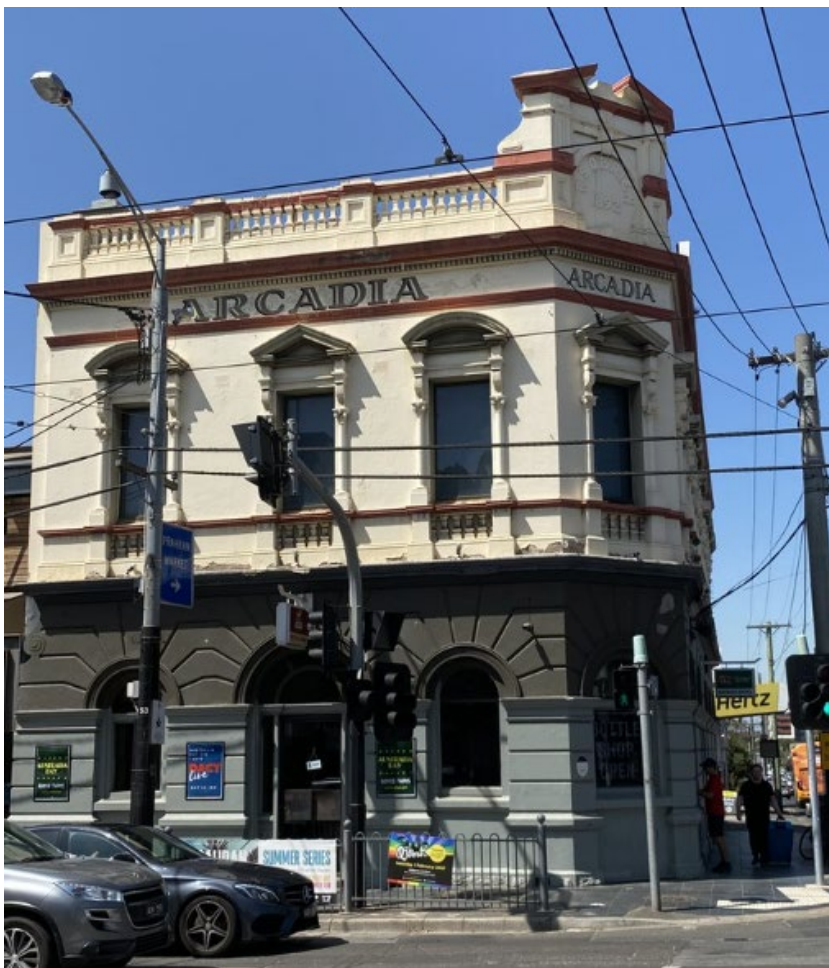
Figure 24. Former South Yarra Hotel at the corner of Toorak Road and Punt Road. (Source: Context, February 2020)
