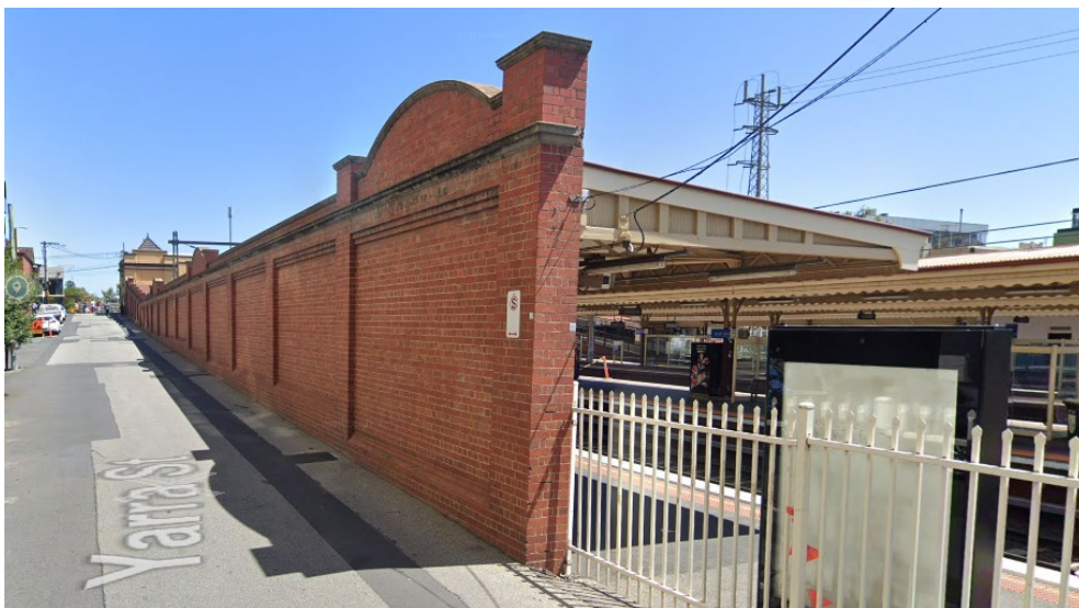
Figure 27. Red face brick wall on the western side of Yarra Street supporting the canopy on platform 6 (Source: Google January 2019)
