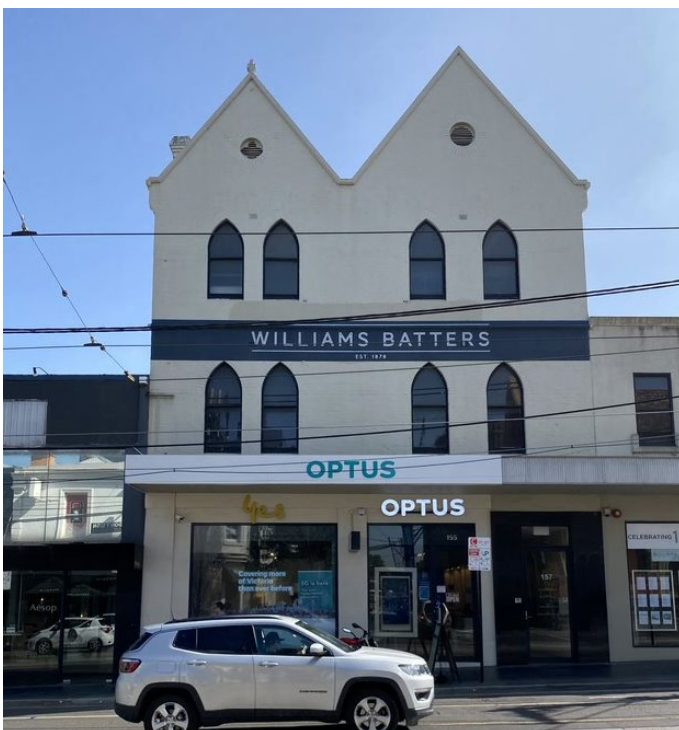
Figure 18. Victorian Gothic building, c.1878 at 155-157 Toorak Road (between Darling Street and Yarra Street). (Source: Context, February 2020)
