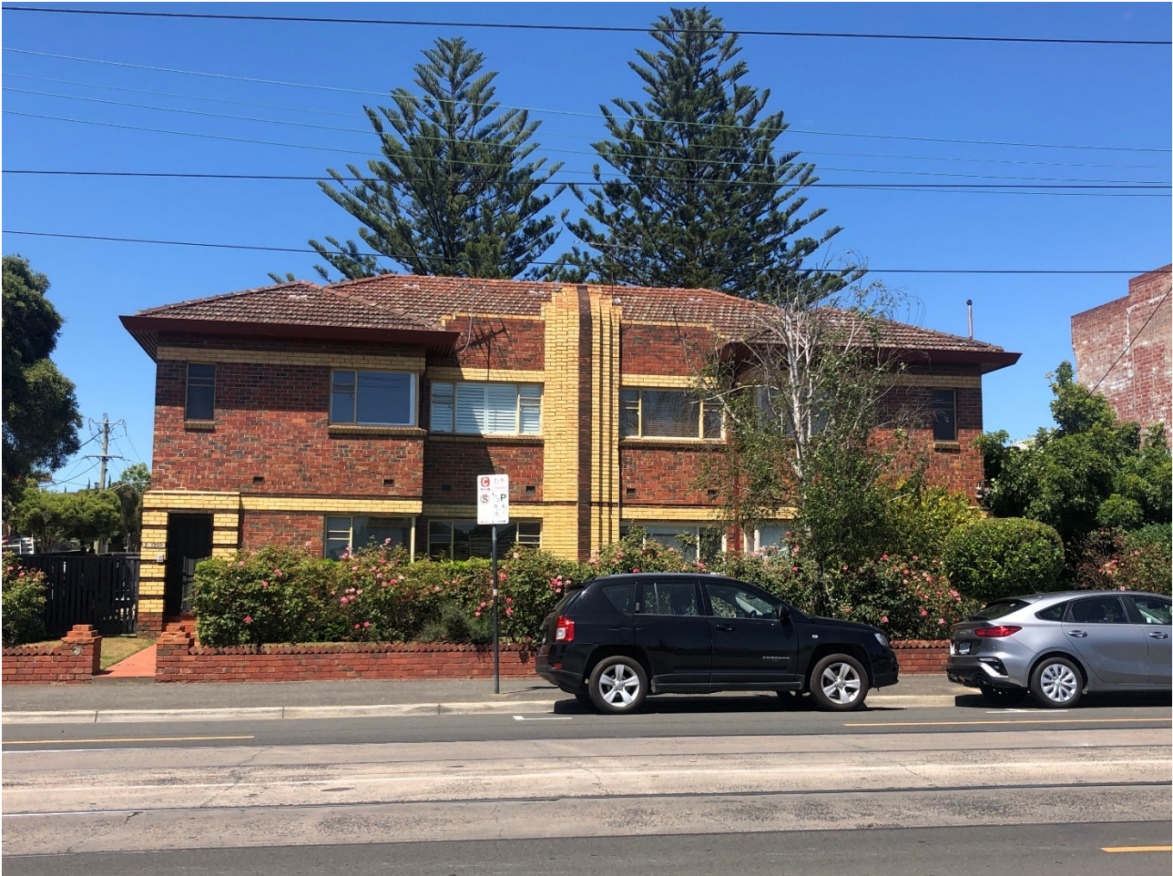
Figure 1. 1298 Malvern Road, Malvern (November 2020)
