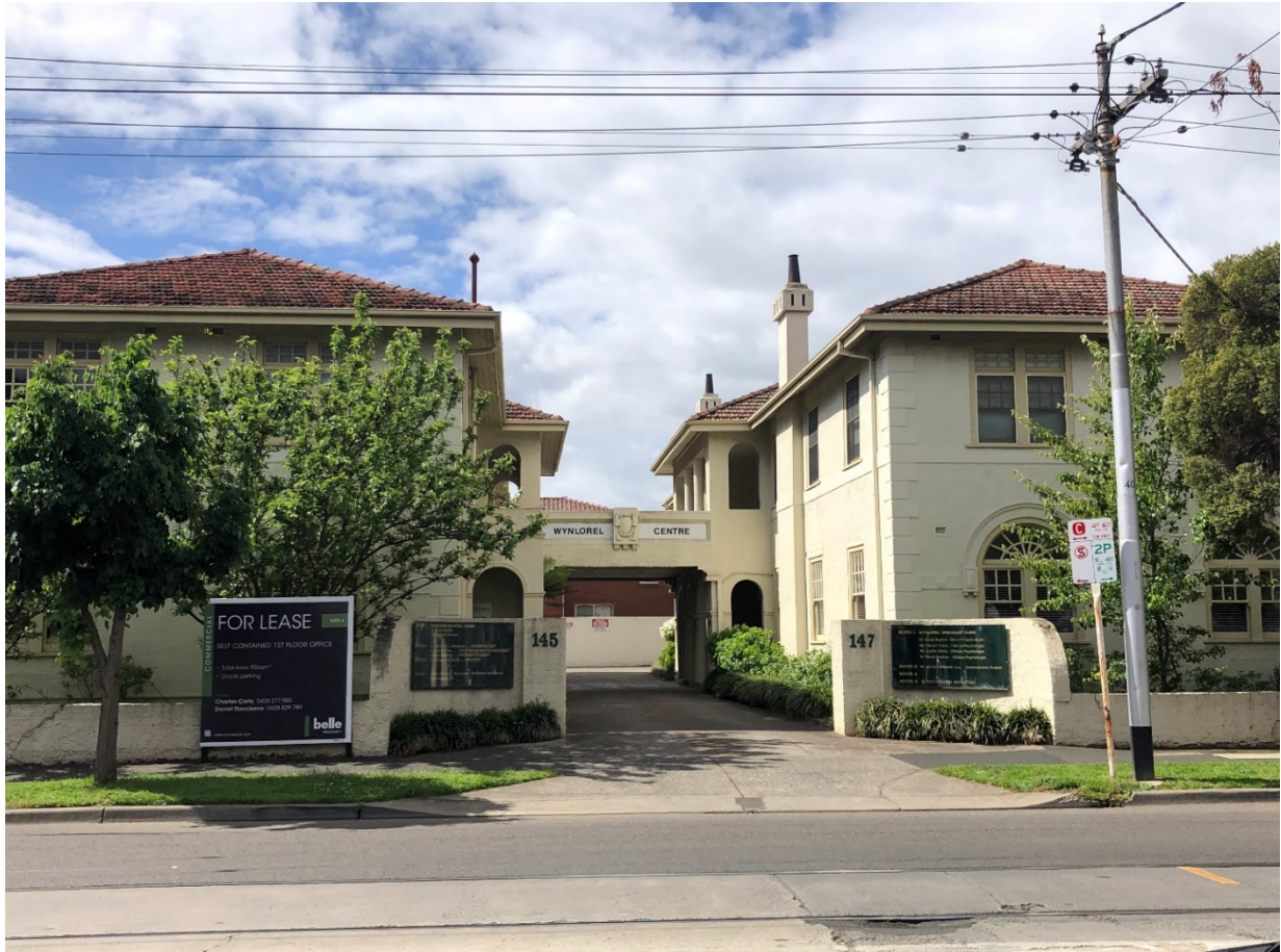
Figure 145 & 147 Wattletree Road, Malvern (southern elevation) (December 2020)
