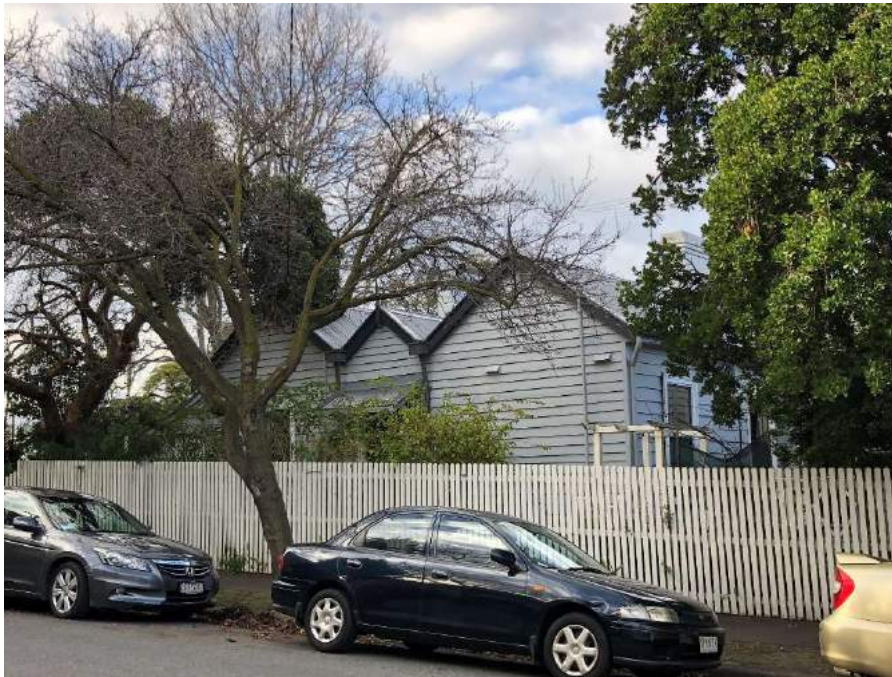
Figure 2. Western elevation to Glendearg Grove (GJM Heritage, July 2020).
