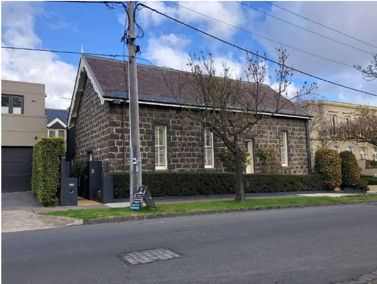
Figure 1.19 Mayfield Avenue (GJM Heritage, July 2020).
