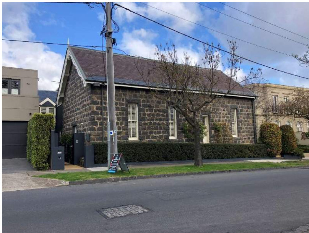
Figure 1.19 Mayfield Avenue (GJM Heritage, July 2020).
