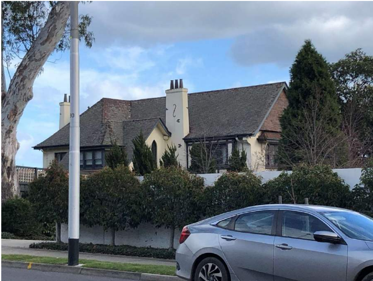
Figure 1. 429 Glenferrie Road, Malvern (GJM Heritage, July 2020).
