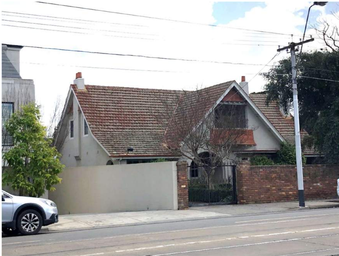
Figure 1. 333 Glenferrie Road, Malvern (GJM Heritage, July 2020).
