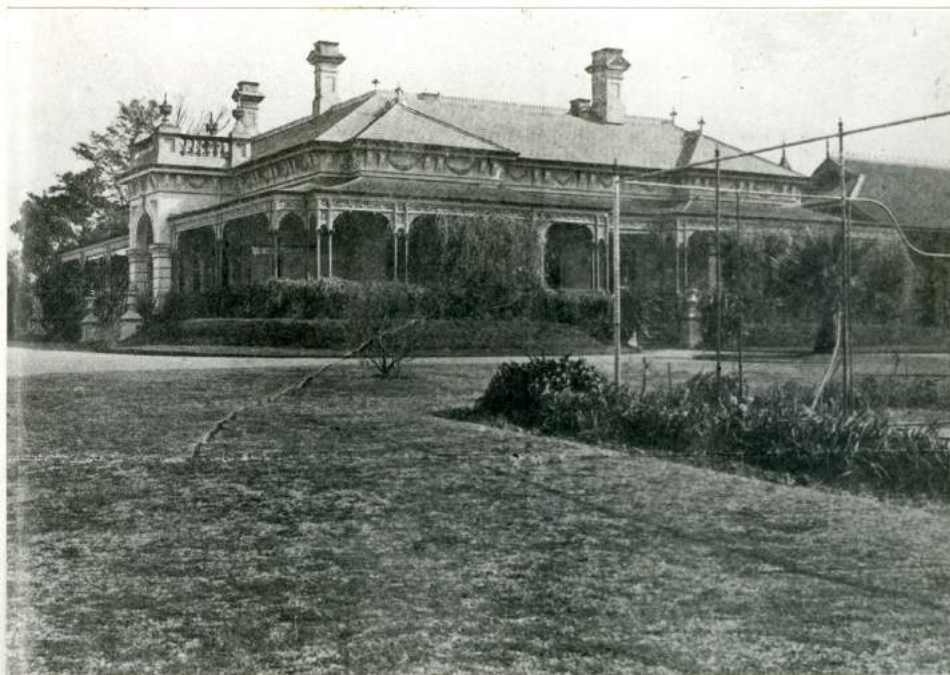
Figure 6. View of the east elevation of Northbrook, 1929 (Source: SHC MP358)
