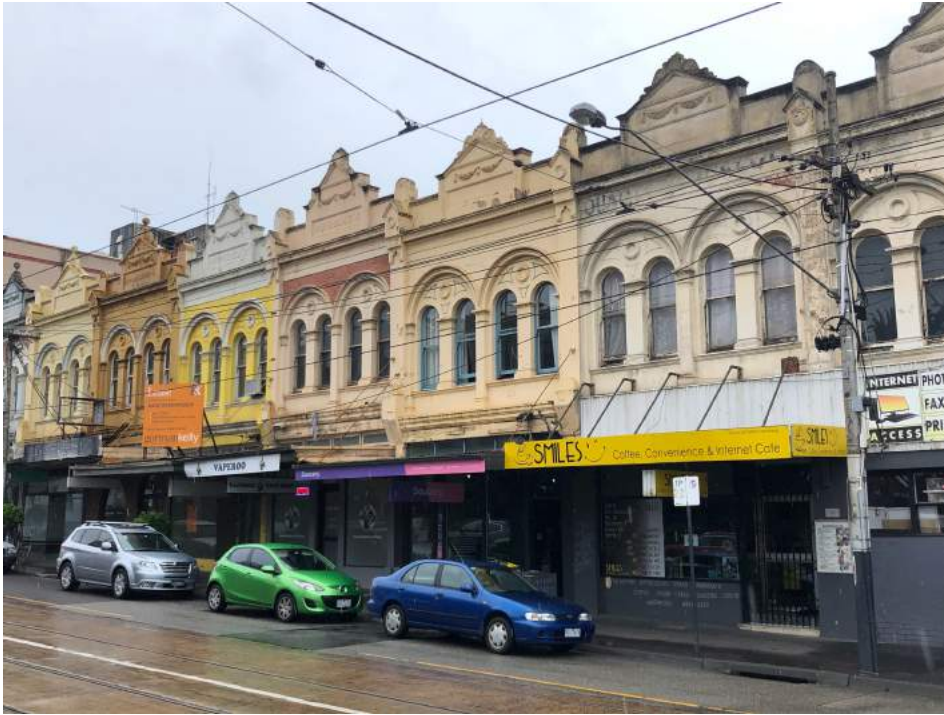
Figure 7. Pepperell's Building, 13-25 Glenferrie Road
