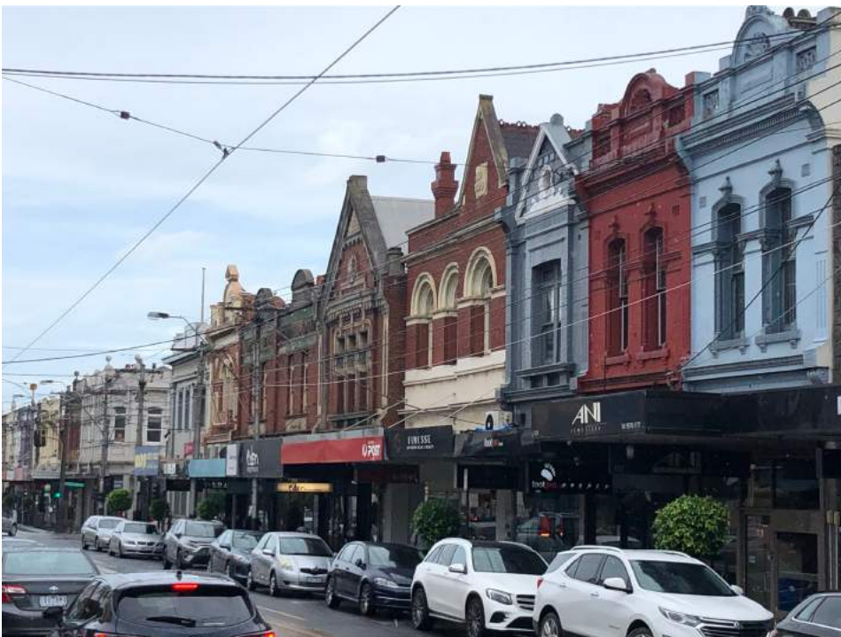
Figure 6. Western side of Glenferrie Road, north of Wattletree Road
