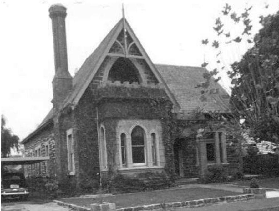
Figure 8. House, 1 Sorrett Avenue, 1963. (Source: SHC MP12230)
