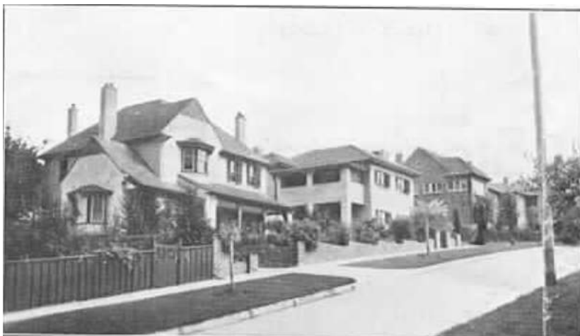
Figure 5. Photo dated c1935, looking north at 3-9 Henderson Avenue (SHC, MP5286).
