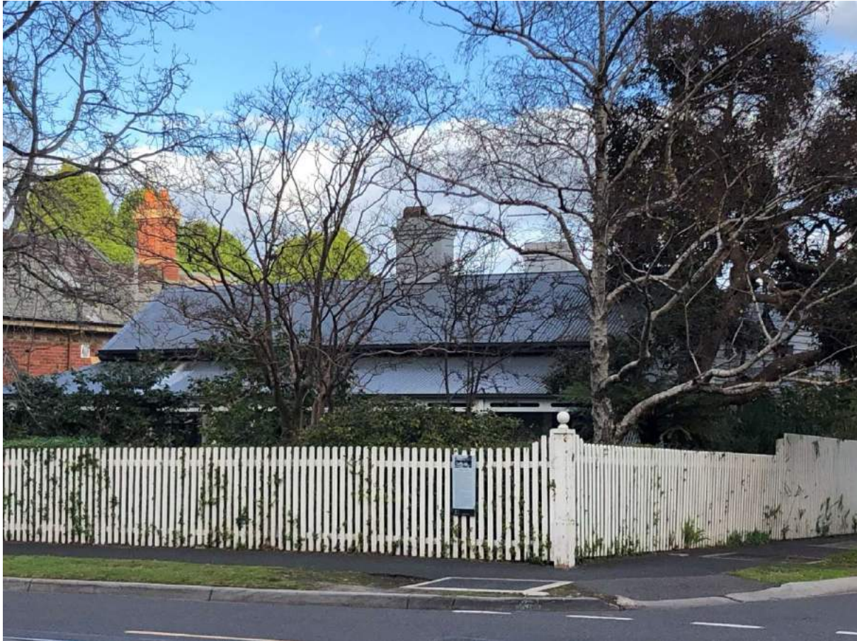
Figure 1. 196 Wattletree Road, Malvern (GJM Heritage, July 2020)
