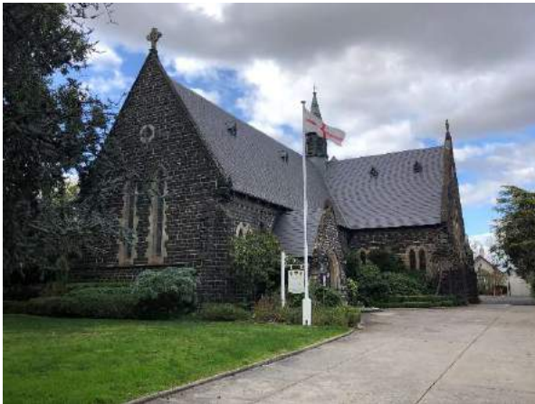
Figure 1. St George's Anglican Church (GJM Heritage, July 2020).
