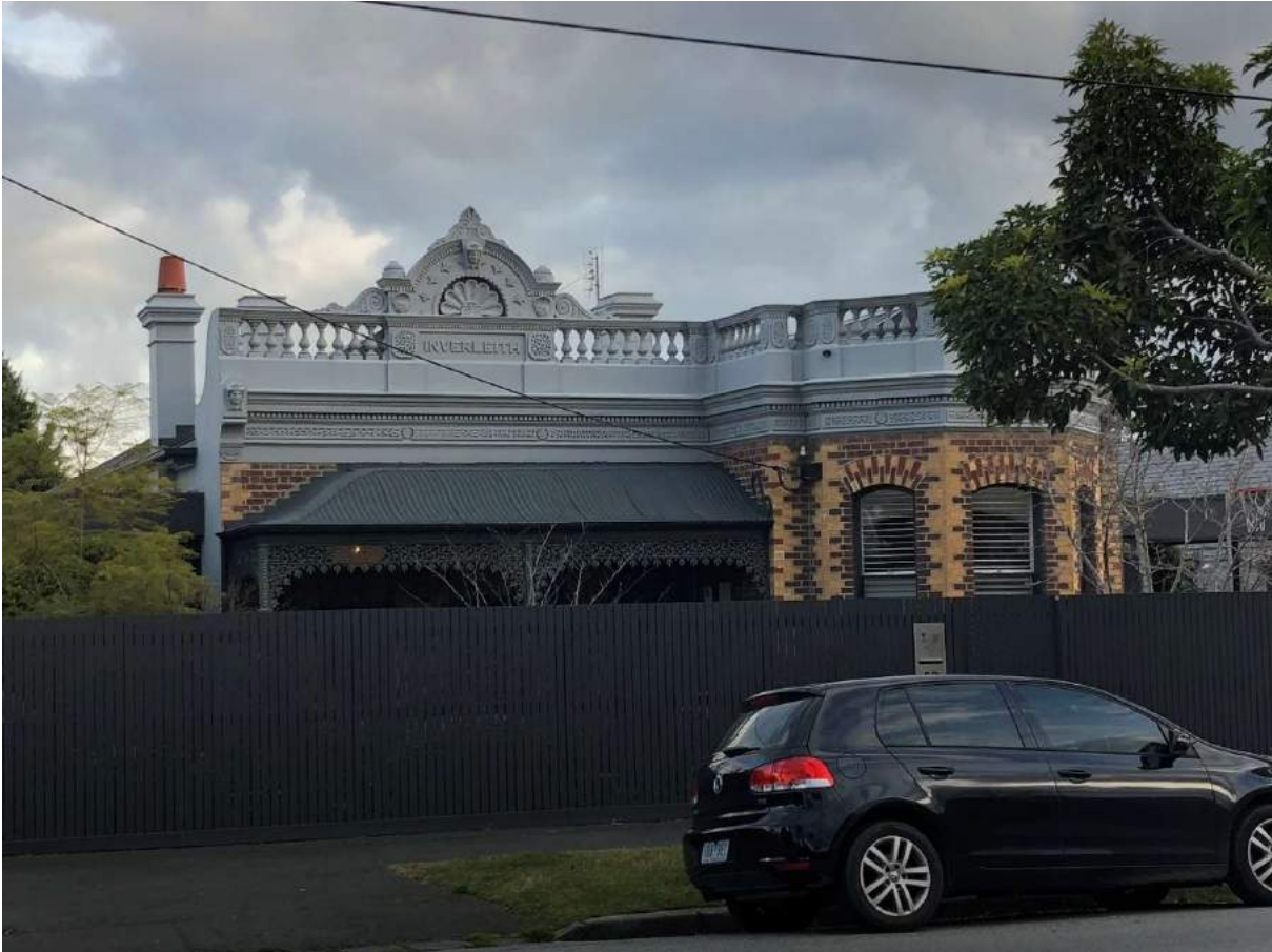
Figure 1. 50 Stanhope Street, Malvern (GJM Heritage, July 2020)
