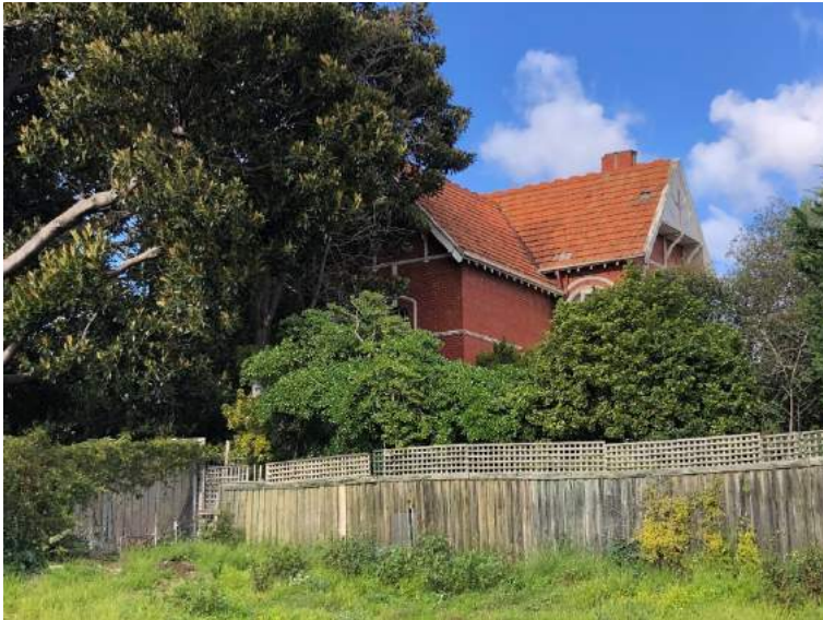
Figures 1. 6 Mayfield Avenue, Malvern: the main (north and west) elevations of the house (GJM Heritage, July 2020).
