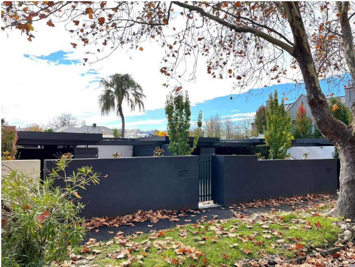
Figure 1. 11-13 Sorrett Avenue, Malvern (GJM Heritage, May 2021).
