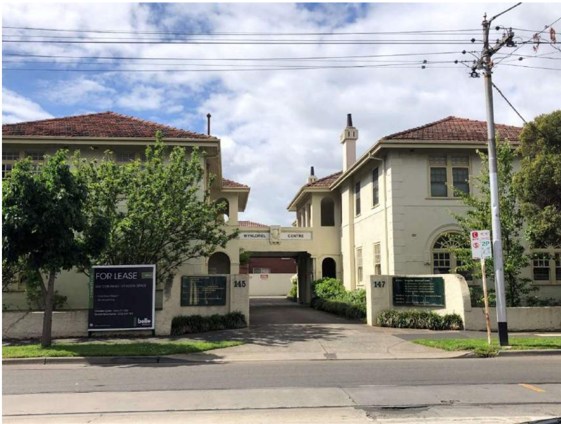
Figure 1. 145 & 147 Wattletree Road, Malvern (southern elevation) (GJM Heritage, November 2020).
