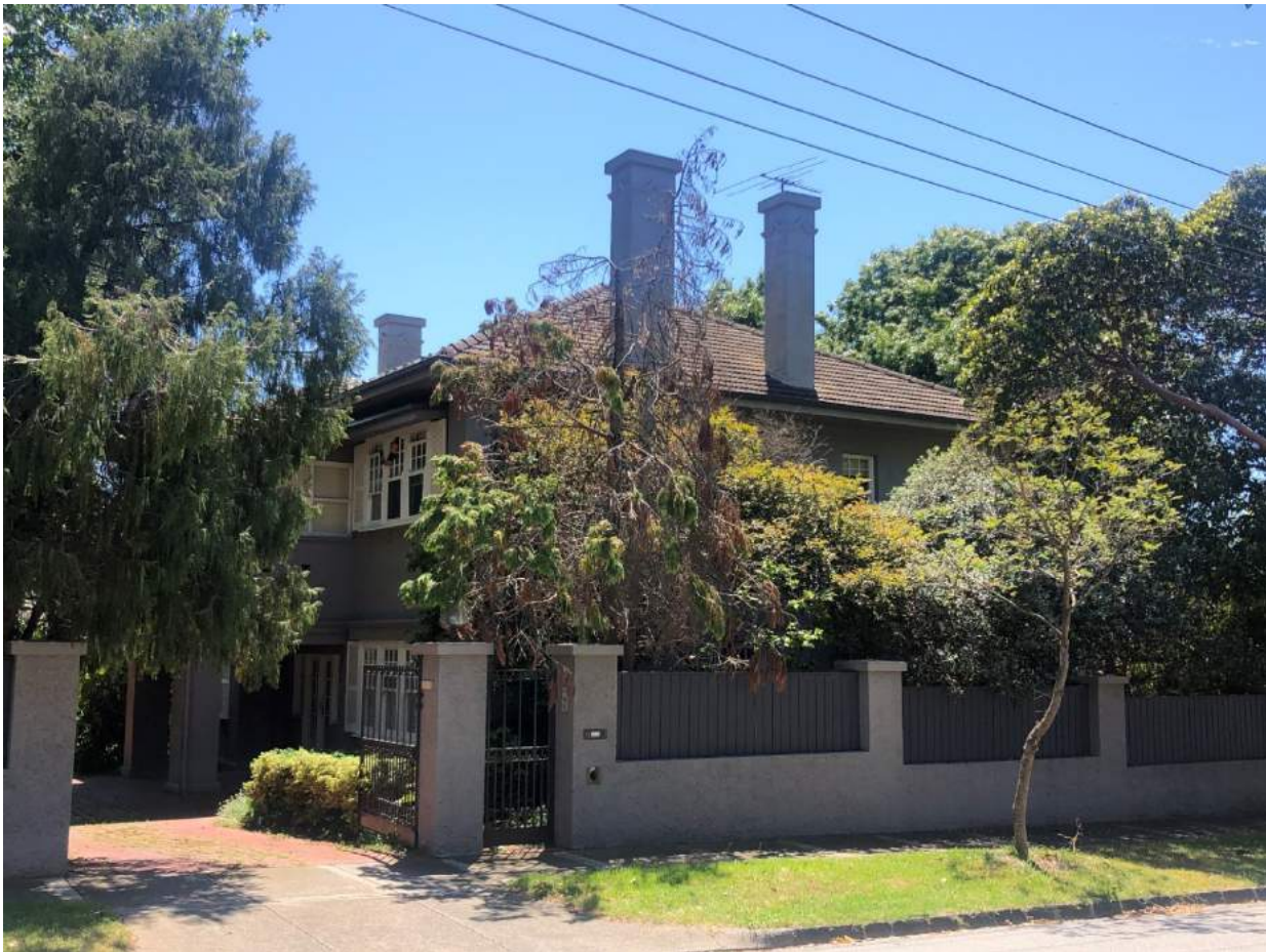
Figure 1. 328 Glenferrie Road, Malvern (GJM Heritage, November 2020).
