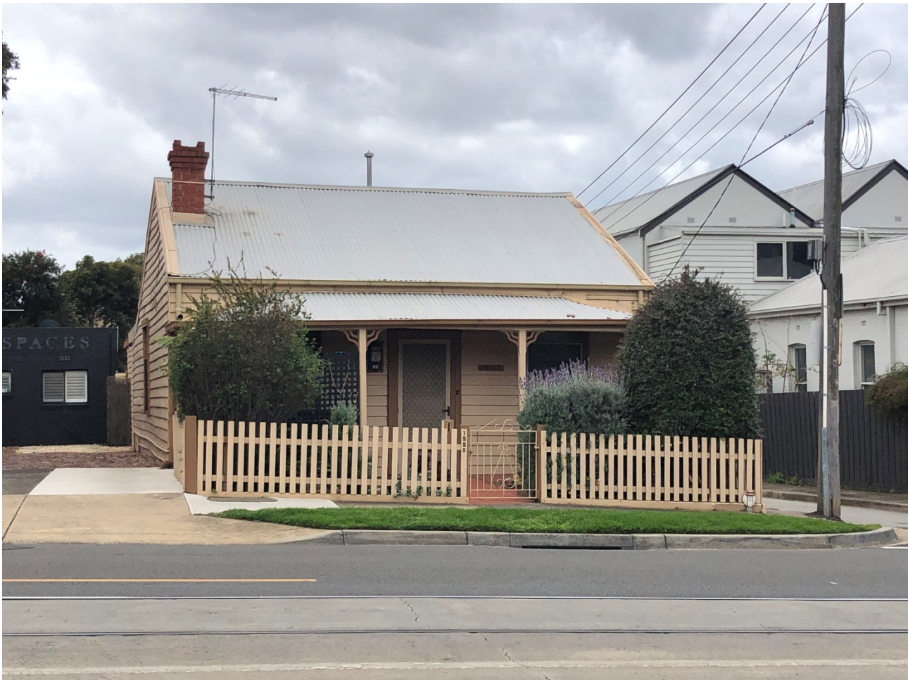
Figure 1. 1225 Malvern Road, Malvern (GJM Heritage, December 2020).
