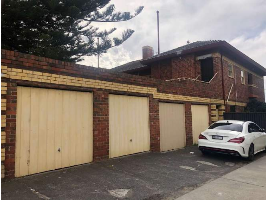
Figure 5. Garages to Shaftesbury Avenue (GJM Heritage, November 2020)
