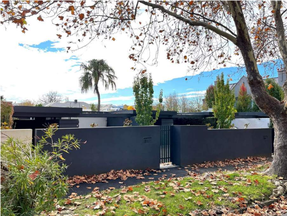
Figure 1. 11-13 Sorrett Avenue, Malvern (May 2021)
