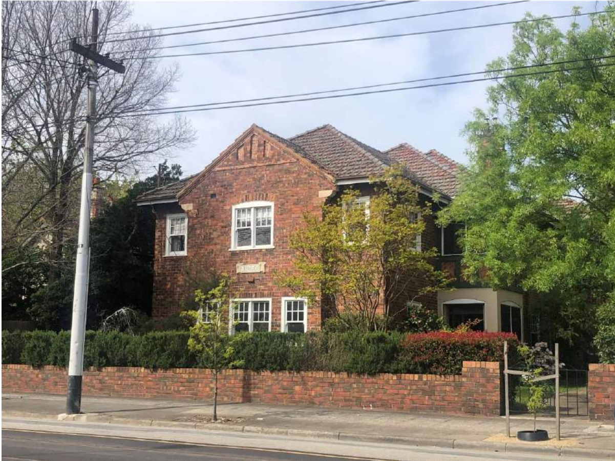
Figure 1. 298 Glenferrie Road, Malvern (December 2020)
