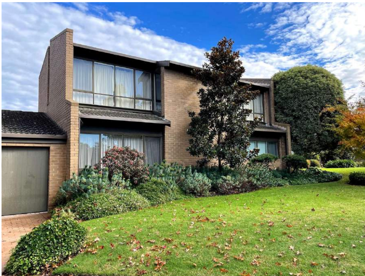
Figure 1. Part of the Hamilton Close Cluster Housing at 1 & 9 Hamilton Road, Malvern (May 2021)
