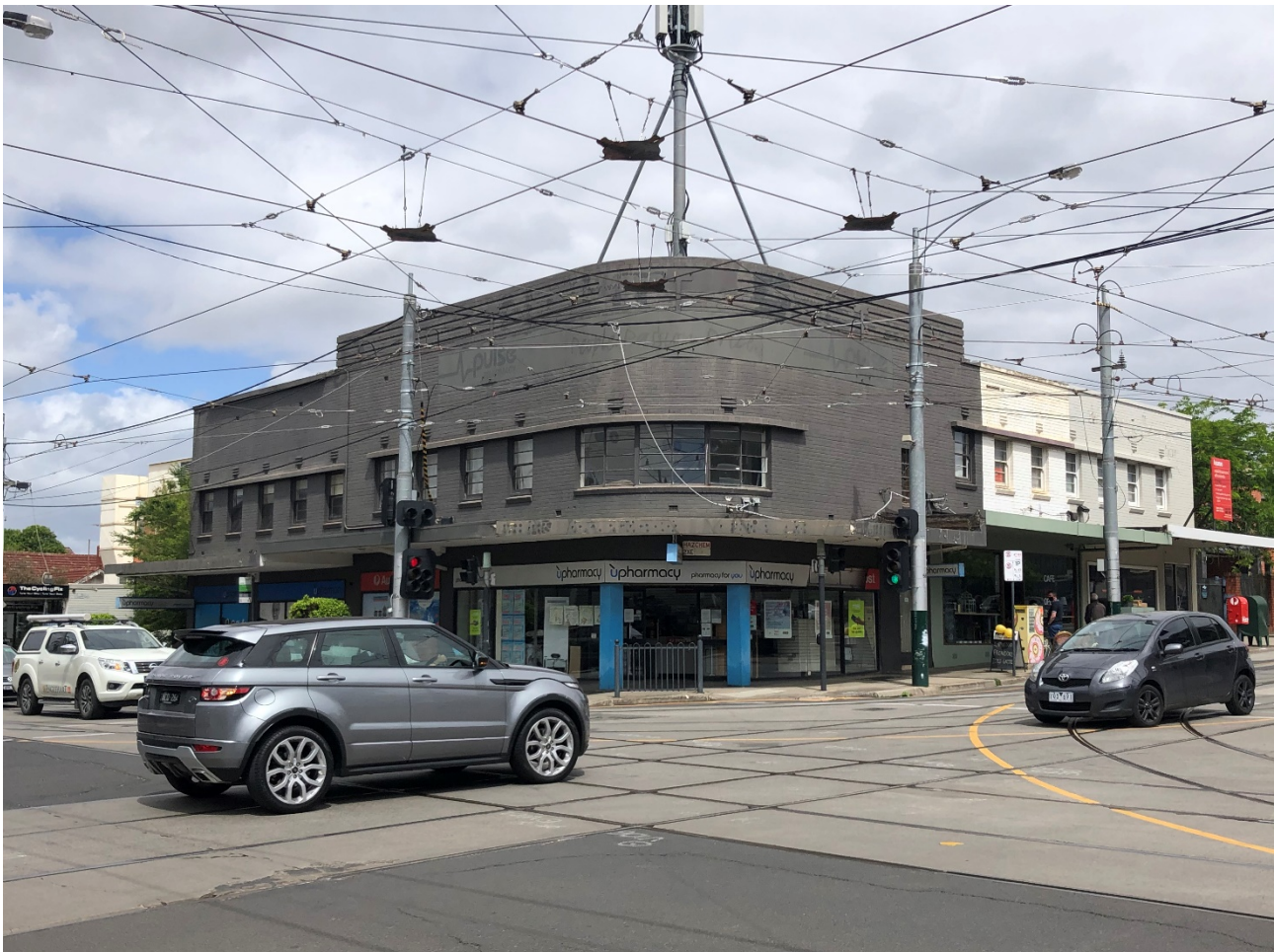
Figure 1. 318-318B Glenferrie Road & 1112-1122 Malvern Road (southern elevation to right, eastern elevation to left), Malvern (GJM Heritage, November 2020).
