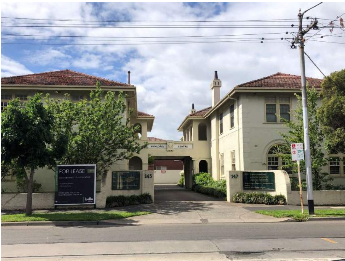
Figure 145 & 147 Wattletree Road, Malvern (southern elevation) (December 2020)
