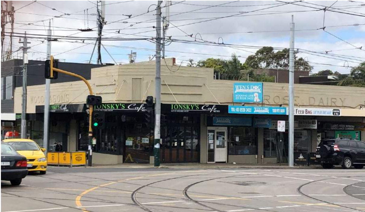
1125-1131 Malvern Road & 320B-320C Glenferrie Road, Malvern (November 2020).
