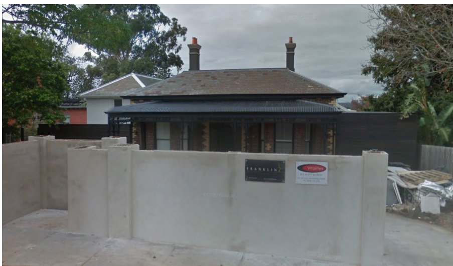
Figure 6. The house at 52 Elizabeth Street, Malvern in 2013 during works (Google Streetview)
