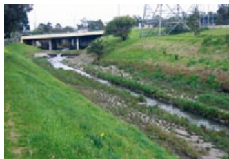
xx View in 2005 of Gardiners Creek near Toorak Road showing the remnant c.1940 bluestone-lined channel. [Context 2005]
