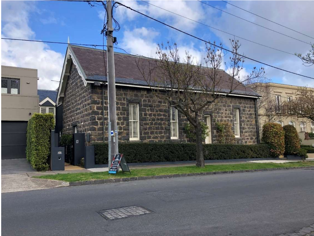
Figure 1.19 Mayfield Avenue (GJM Heritage, July 2020).
