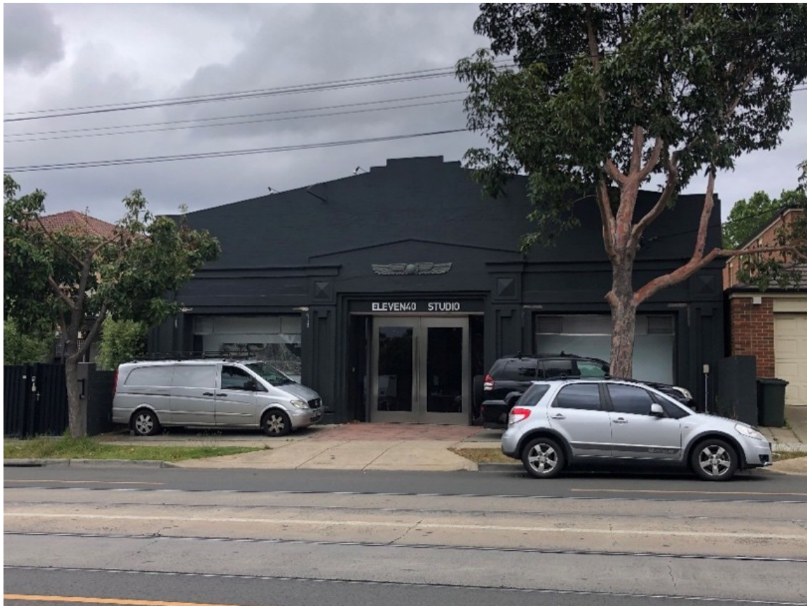
Figure 1. 1140 Malvern Road, Malvern (November 2020)
